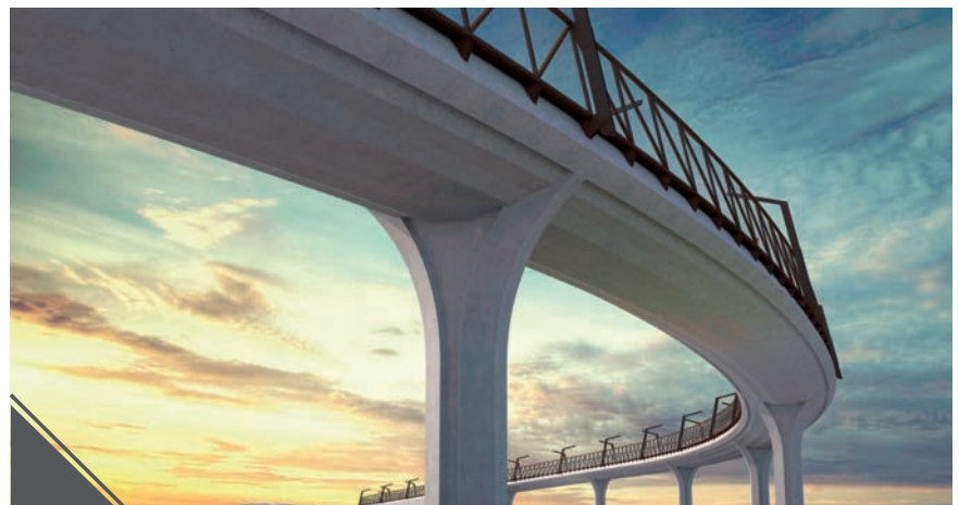
MAINTENANCE ROAD LOOKING WEST (DAYTIME)
