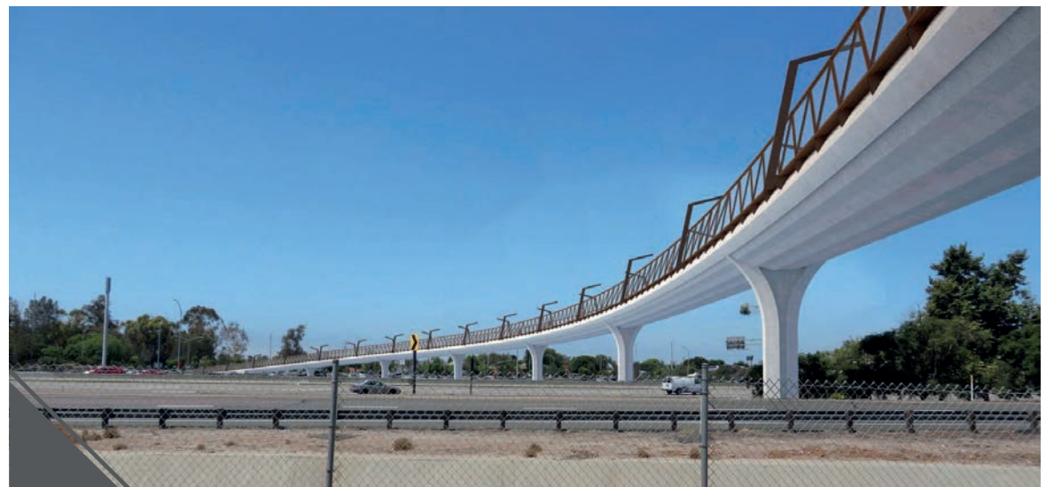
MAINTENANCE ROAD LOOKING NORTHWEST
